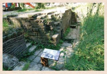
A German concrete bunker at the Bayernwald. It can be seen that the shelter is built roughly flush with the surrounding ground surface, and entered via the trench. Note the construction, individual blocks of concrete having been cast off site and then used like giant bricks cemented together and reinforced with rods. (Author's collection)
