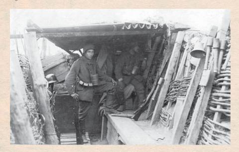
Left: Front line German observation and gas alarm post c.1917. The trench features a sturdy fire step, and revetment of wood and wattle, though the overhead cover is at best splinter and rain proof. One man watches using a concealed periscope with a rifleman on guard. Foreground right is the gas alarm bell, and grenades hung by their belt hooks for convenient close defence. (Author's collection)
