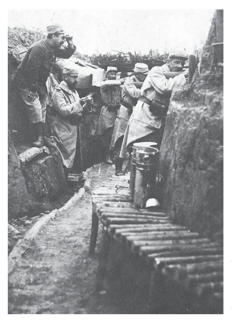
French troops manning a fire trench, 1915. There is a wooden fire step, and the riflemen aim through loops in the parapet rather than over it. The floor of the trench has both a walkway and a separate drainage channel. The cylindrical objects, foreground, are food containers. (Author's collection)
