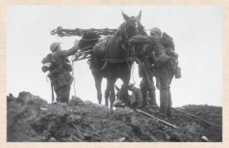
Above: A packhorse, with a gas mask bag secured to his head harness, is loaded with supplies near Pilckem, 31 July 1917. The long items on top of the burden are metal screw pickets to hold barbed wire in place. Screwing in metal pickets was usually quieter than banging in wooden stakes. (IWM Q5717)
