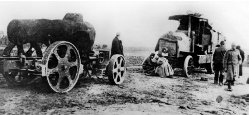
The use of motorised vehicles was still in its infancy in 1915, limited by the unreliability of engines and the lack of adequate roads. Here, a tractor is attached to a 305mm mortar in the Carpathians in 1915. (©2003 Topham Picturepoint)
