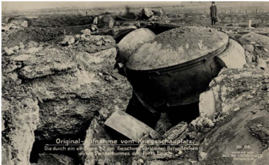
ABOVE: THE CONCRETE ROOF OF A GUN EMPLACEMENT ON ONE OF THE LIÈGE FORTRESSES, DESTROYED BY A GERMAN 420MM SHELL.
