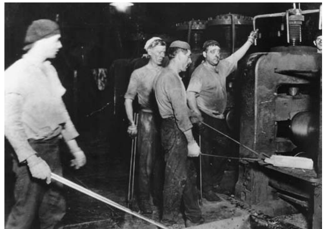
8-9 Workers removing hot steel from the furnace before sending it to the rolling machine.
