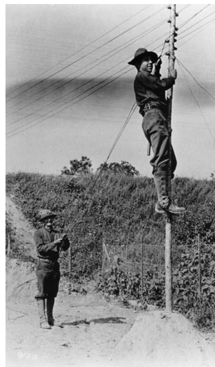
5-25 GI rigging telephone line.
