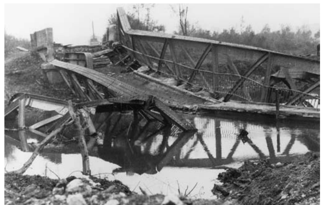
9-26 Bridge across the Aire River blown up by retreating Germans. Note the temporary footbridge built by engineers of the 1st Division. Floville, France, October 1918.
