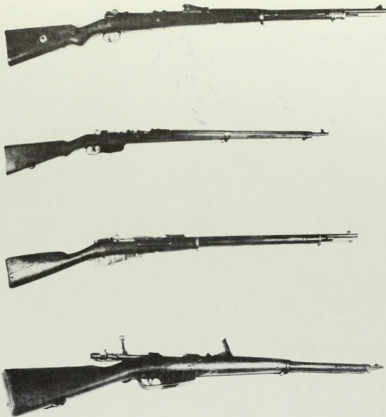
The principal shoulder weapons of World War I, from top to bottom: German 7.92mm Mauser, Model 1898; Austrian 8mm Mannlicher, Model 1895; Russian 7.62mm Moisin-Nagant (or "Three Line Nagant"), Model 1891; and Italian 6.5mm Mannlicher-Carcano, Model 1891 (three-quarter right view, with rear sight leaf up and bolt open).
