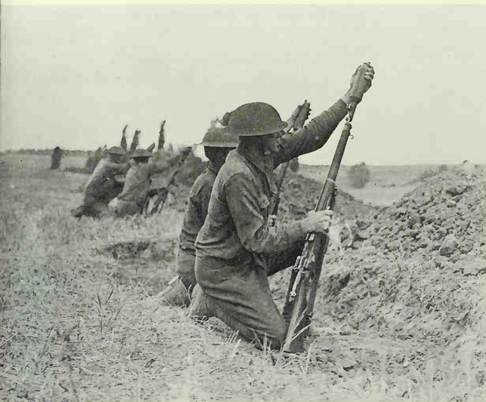
U.S. troops attaching the tromblon , a discharger cup invented by the French, to the muzzles of their rifles in preparation for firing grenades. The cup was a great improvement over the old percussion-type rifle grenade with steel tail rod that sometimes damaged the rifle.
