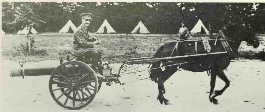
A 240mm (9.45-inch) trench mortar mounted for pony cart transport at Saint-Pol Trench Mortar School, July, 1917. The original of this mortar was designed by the Société Batignolles and weighed more than 3 tons. Later versions were manufactured in England and the U.S. Ranges varied from 1,200 to more than 2,000 yards with shells weighing from 150 to about 200 pounds.
