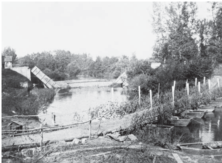
A pontoon bridge, assembled by Royal Engineers of I Corps, spans the River Aisne. The original bridge, destroyed by the retreating Germans, is visible to the rear.
