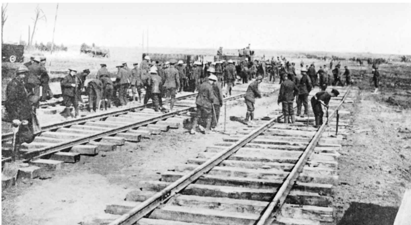
Laying track to bring up supplies for the ongoing offensive. 331GP
