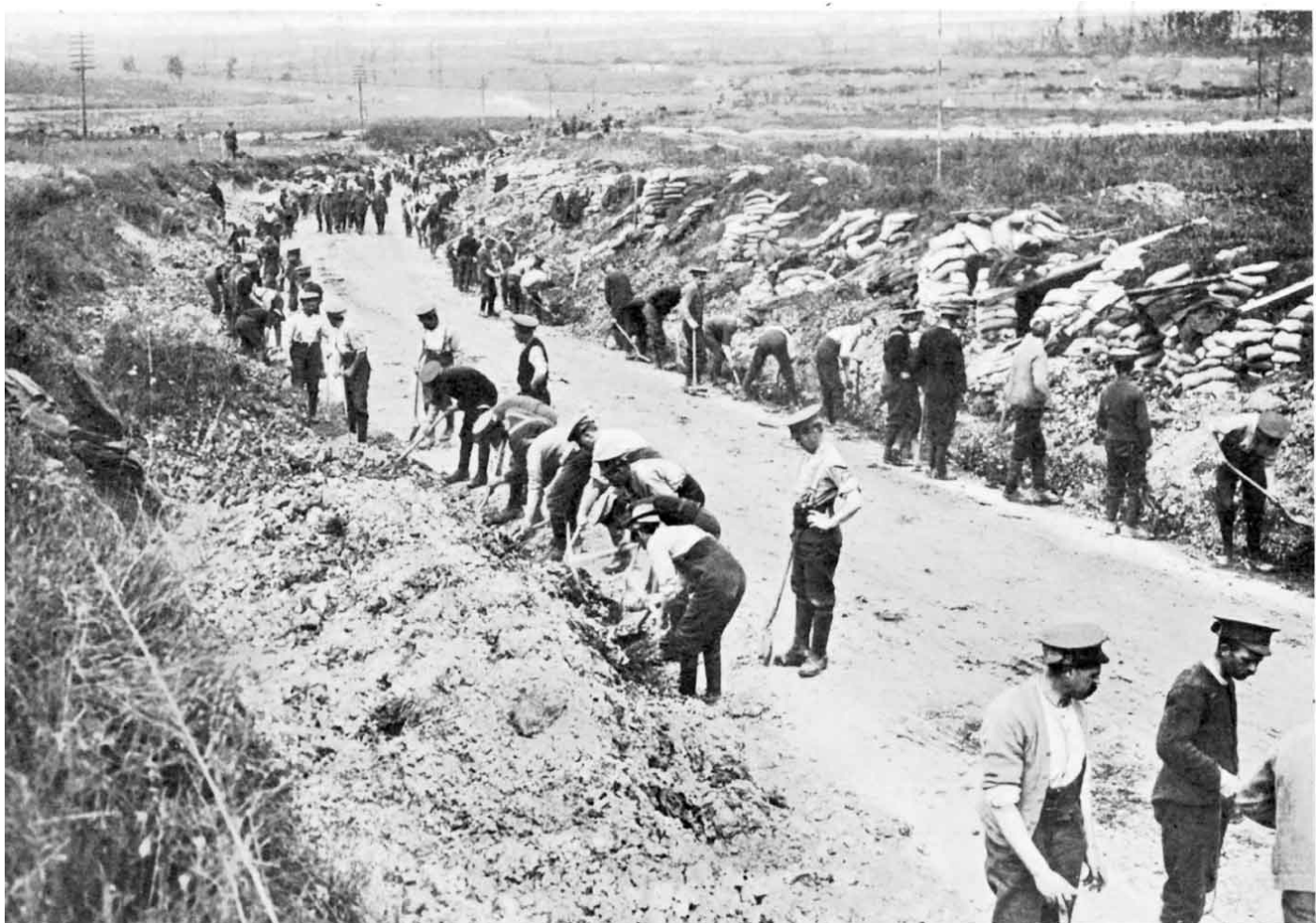
Constant work repairing and widening roads on the Somme. 73BP
