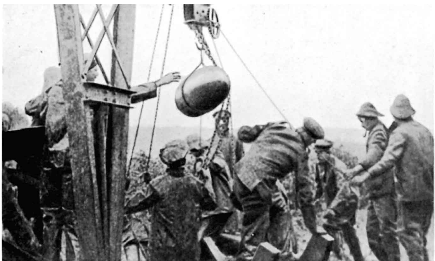
Preparing to load a 15-inch howitzer using a chain hoist system to lift the shells. It could throw a 1,400 lb heavy shell six miles and some considered it hardly worth all the labour and time it took to move and emplace these very heavy guns.
