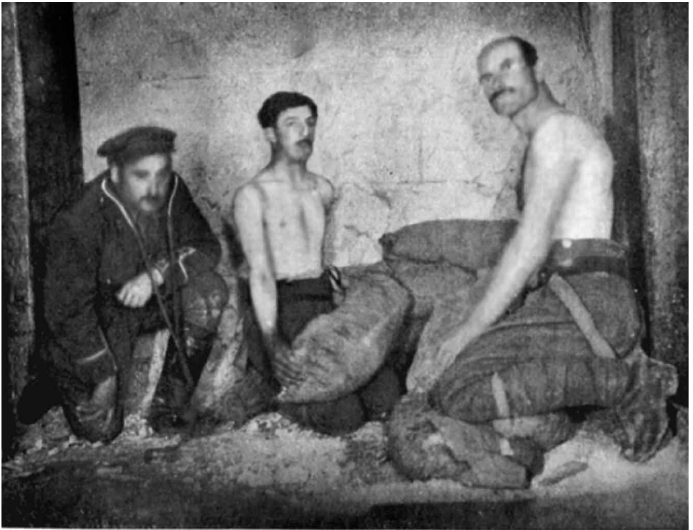
Men of a Royal Engineers Tunnelling Company deep underground beneath the chalking soil of the Somme laying an explosive charge. The officer with the instrument called the geophone is listening for any sounds that would warn of Germans digging a counter-mine called a camouflet . 232GP
