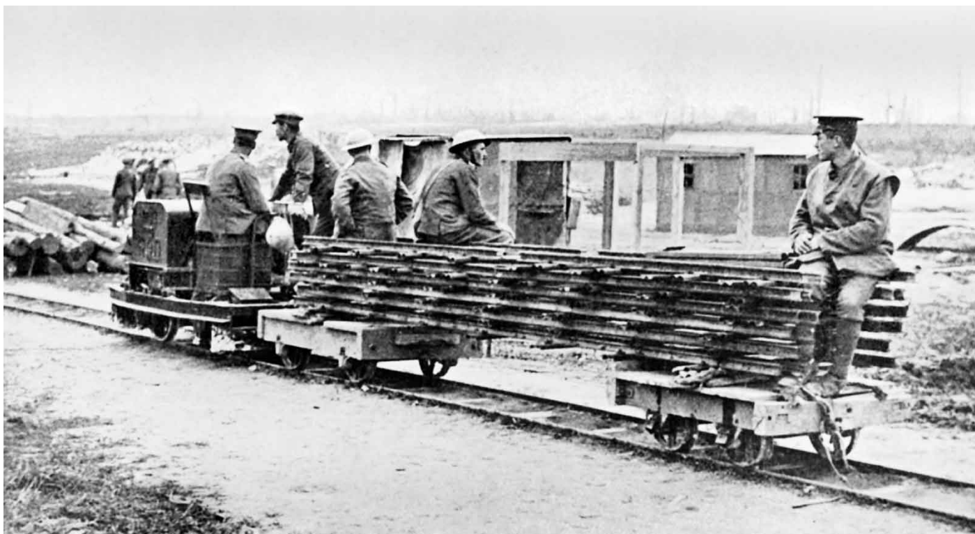
A 20 hp Simplex petrol tractor moving pre-fabricated track panels. 338GP
