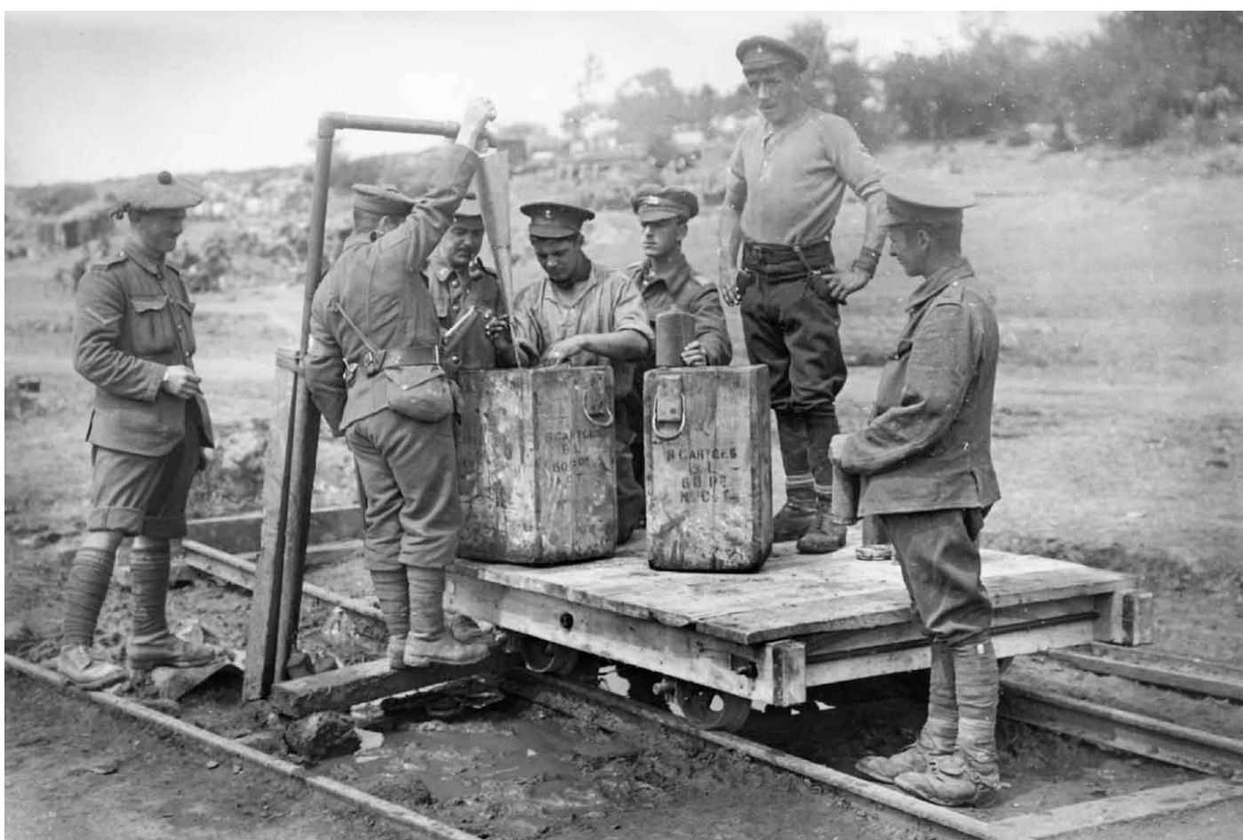
Underground pipeline bringing water to a narrow gauge rail line. 1 GP/W021
