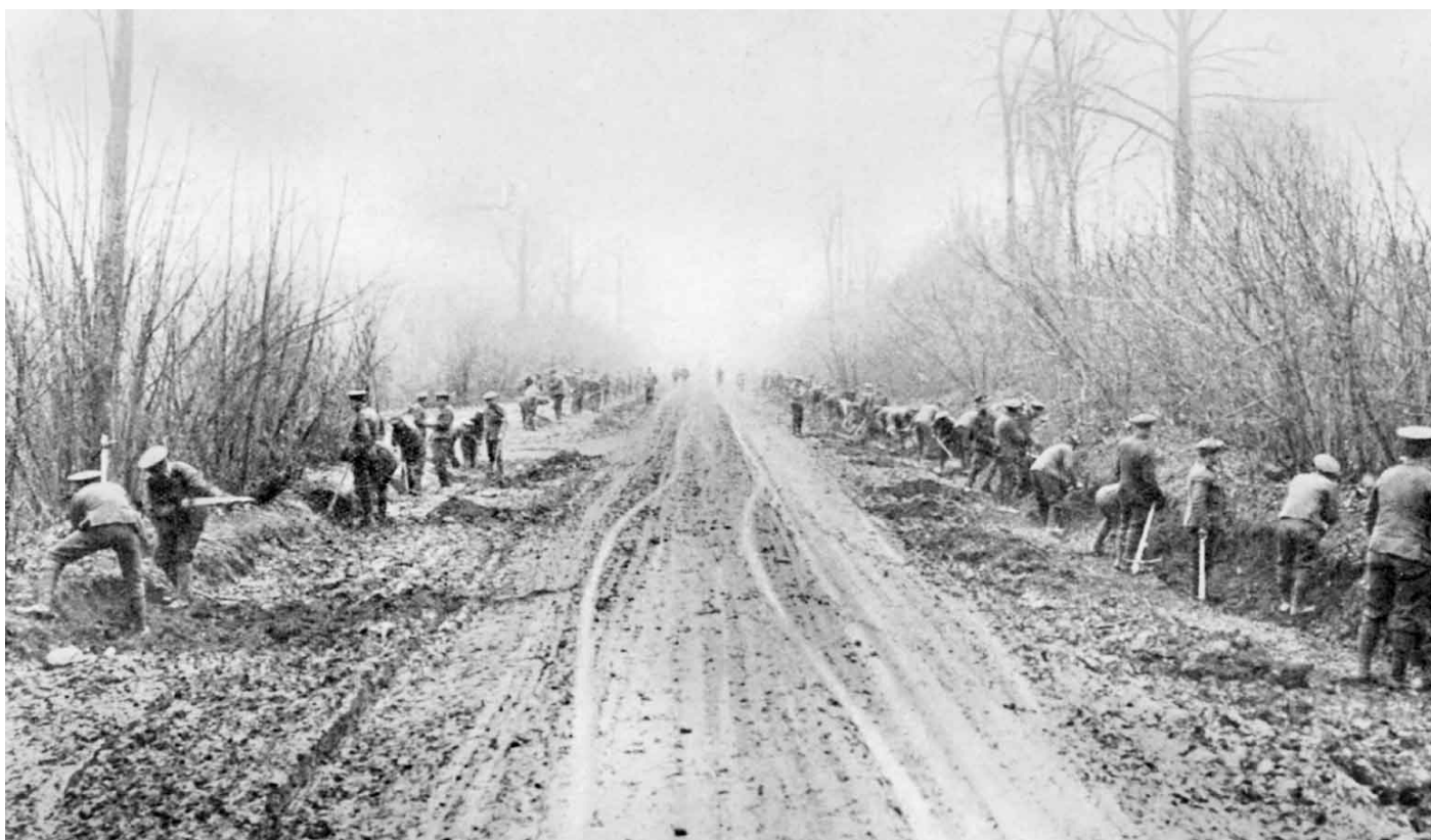
Pioneers digging drainage ditches alongside a supply road. 68BP
