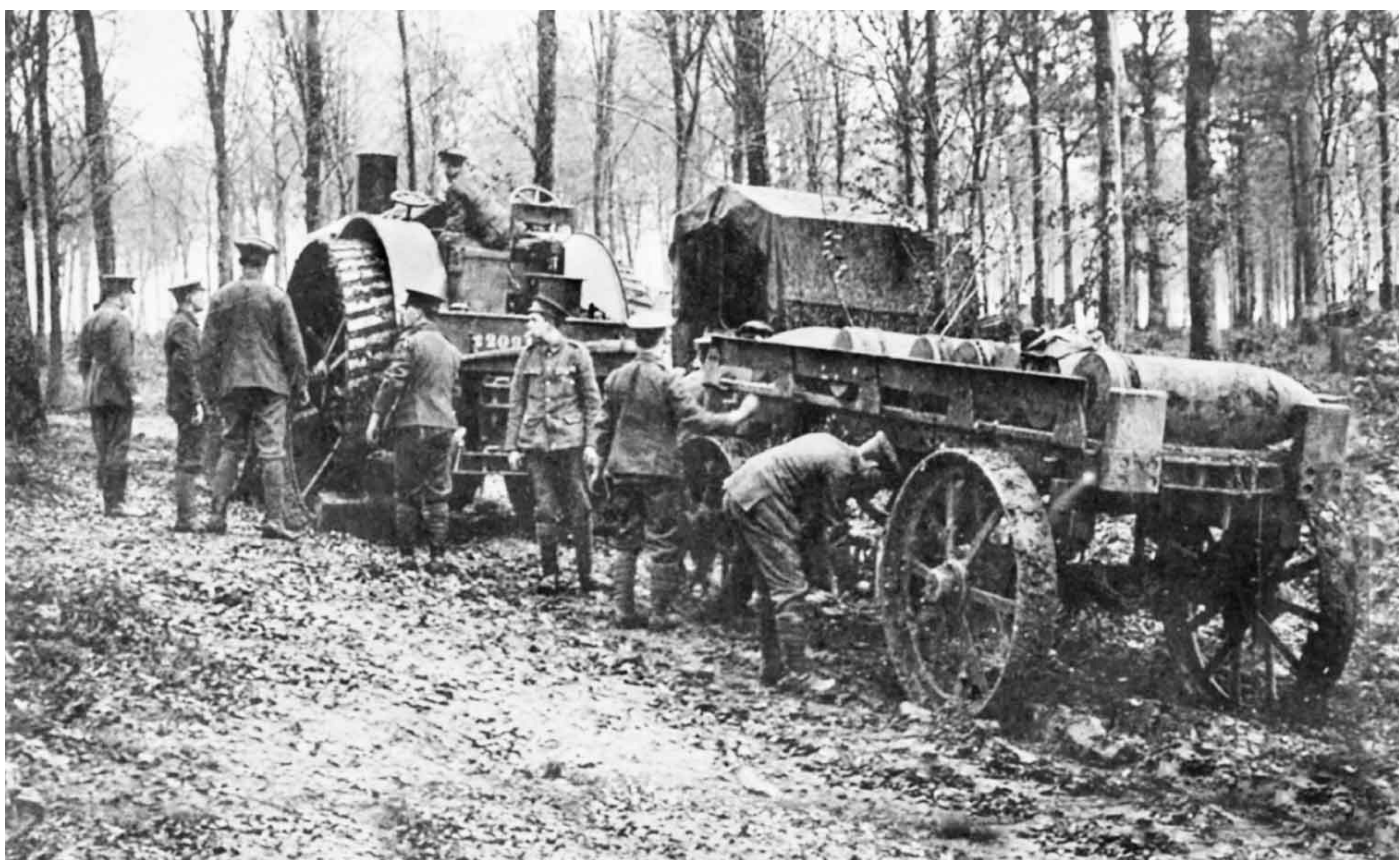
A six-cylinder Daimler engine tractor hauling ammunition. 375GP
